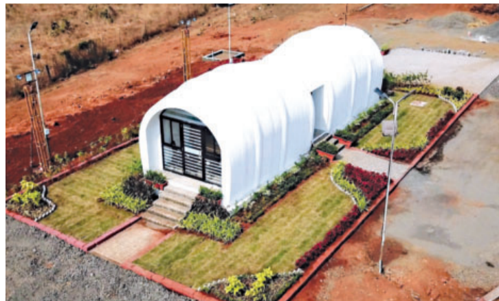
Godrej and Boyce built a 48-square-metre office, named "The Cocoon", in 40 hours using 3D printing
