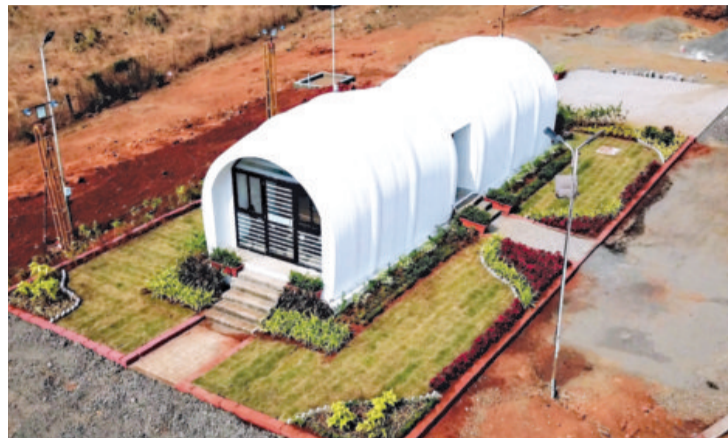
Godrej and Boyce built a 48-square-metre office, named "The Cocoon", in 40 hours using 3D printing
